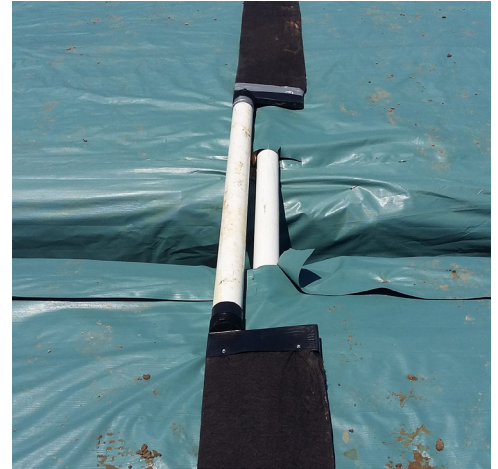
TerraVent connection over footing
